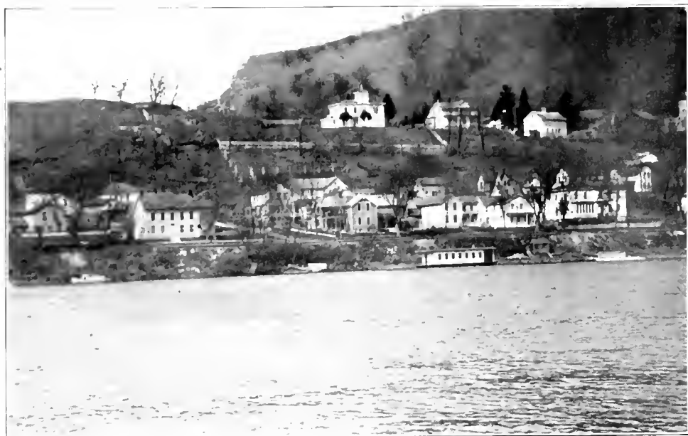
RIVER STREET, LANSING
